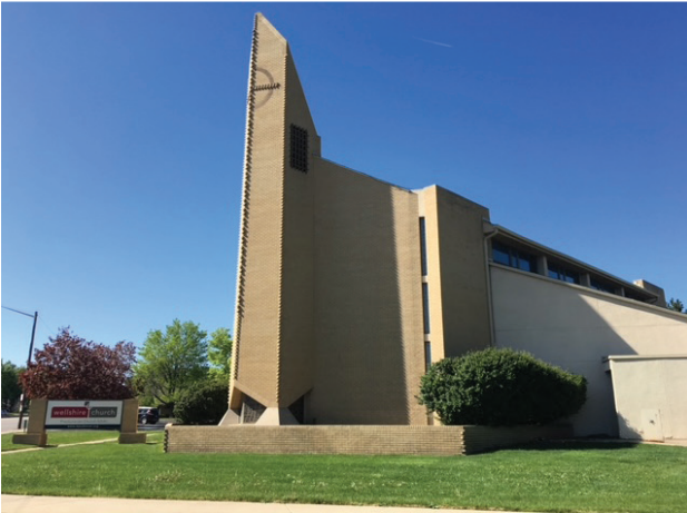
Wellshire Presbyterian Church - Denver, CO - extensive renovations
